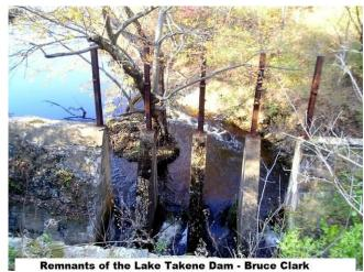
The dam was constructed following a "barrage" design, and consisted of four side-by-side concrete piers with gates that could be opened or closed to regulate the depth of the lake. The remnants of the dam are still visible from the top of the bridge (which is now part of the Patriot's Path network of hiking trails).
