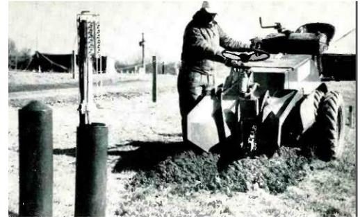
Cable terminals and cable terminal housings (left) and trencher for burying distribution cables were observed.
