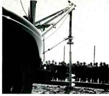
Engineers watch front mounted hydraulic pole digger in operation
