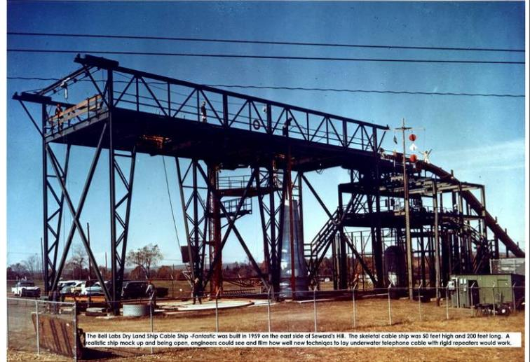
Bell Labs decided to build a skeletal mock up of a full size cable ship at Chester to allow the testing and filming of the many possible configurations and procedures for laying cable and repeaters. The model was called the Bell Labs Dry Land Cable Ship (BLDLC), nicknamed “Fantastic” and was 50' high and 200' long. It was anchored to the side of Seward's Hill. A test is
