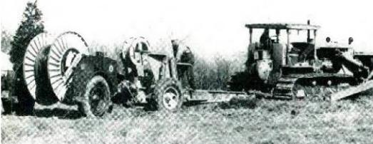
Caterpillar tractor, cable plow unit, and hydraulic cable reel trailer used in laying underground cable.
