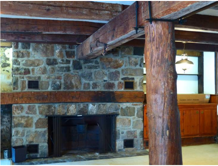
1st floor fireplace, tree trunk supports, and beams
